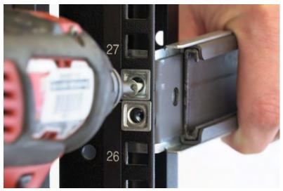
Install the second screw. Make sure the outer member didn't slide during install. If so, loosen screws and readjust.
