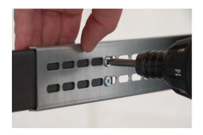
Tighten both screws with screwdriver and repeat on the opposite side.
